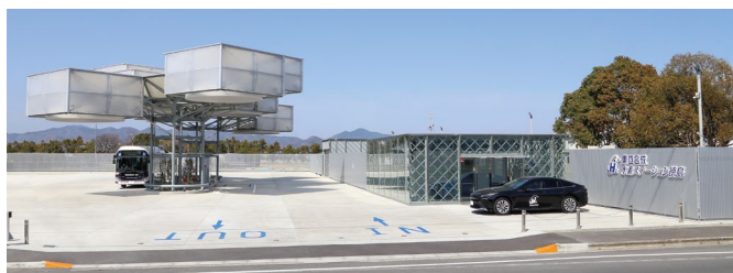
Toagosei Hydrogen Station Tokushima
