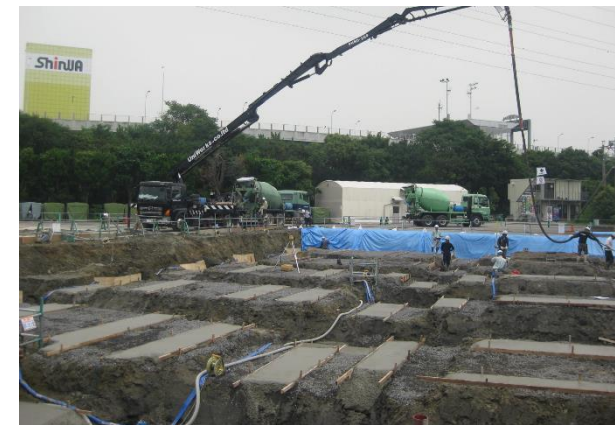
Aronkasei Nagoya Plant Construction of a new building for injection molding-blending
