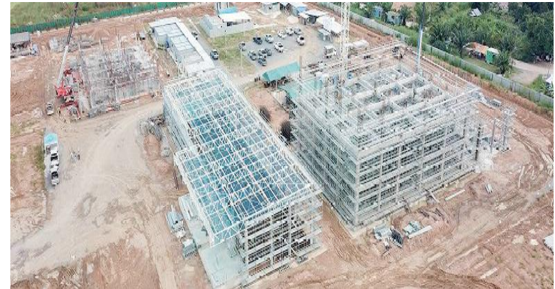
New Thailand plant under speedy construction
