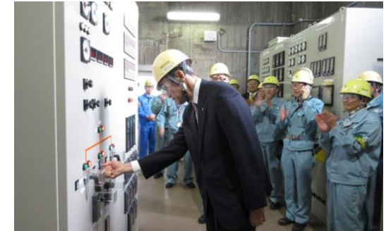
November 2017 - Powering up the new facilities
