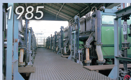
The electrolysis equipment of the Nagoya Plant is changed to the ion exchange membrane method.
