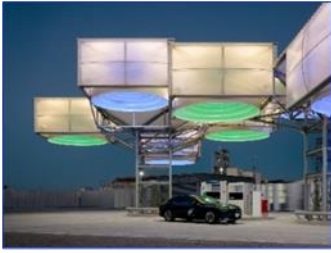
Toagosei Hydrogen Station Tokushima
