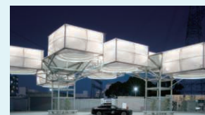
Toagosei Hydrogen Station Tokushima
