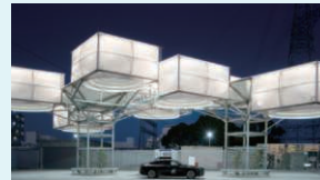
Toagosei Hydrogen Station Tokushima
