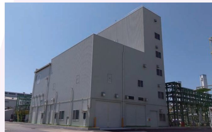
New high-purity liquefied hydrogen chloride facilities of the Yokohama Plant
